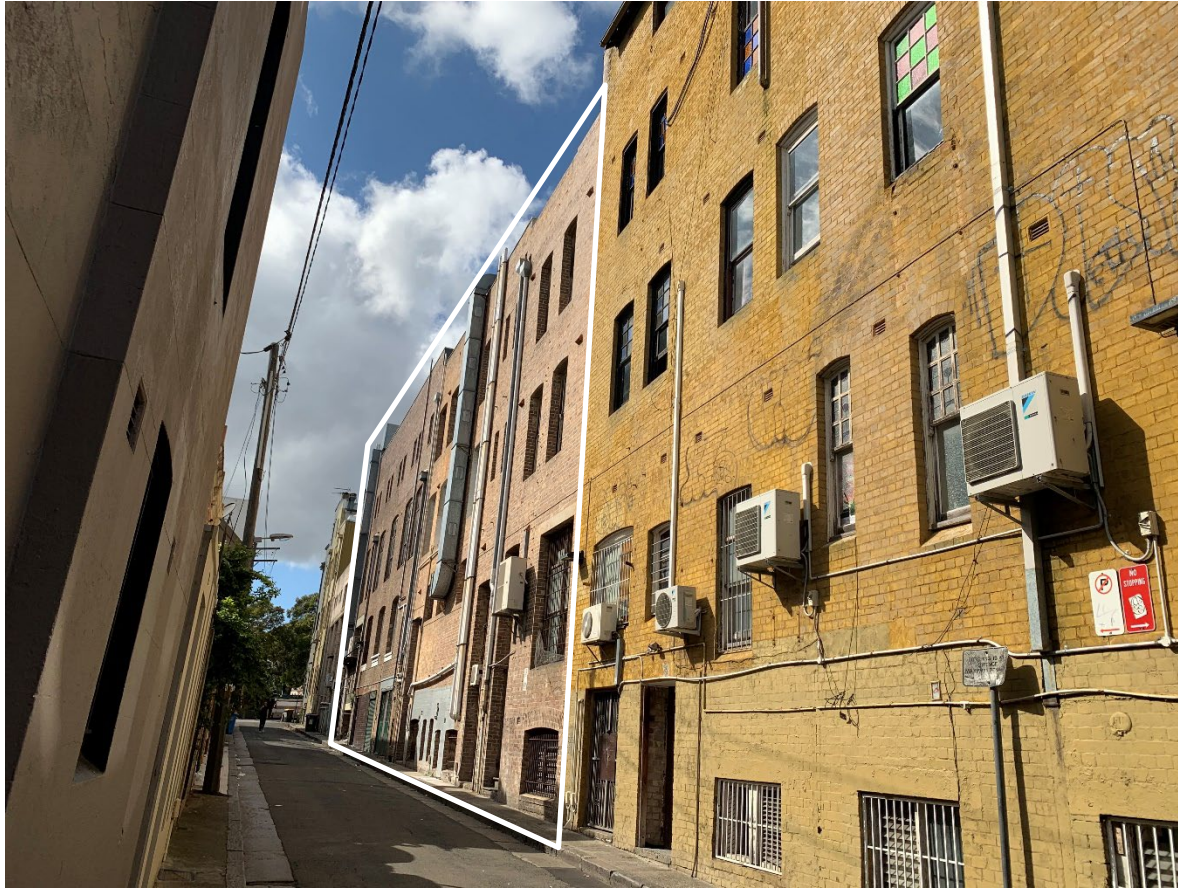
Site viewed from Foley Street
